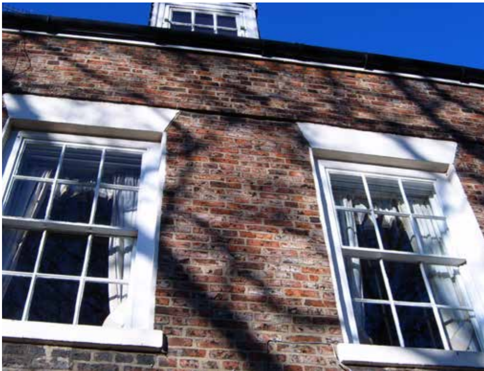
EXAMPLES OF THE EXISTING TIMBER SASH WINDOWS
