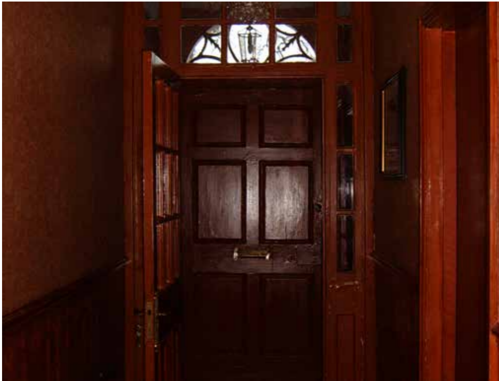
INTERNAL VIEW OF THE EXISTING LOBBY AT THE MAIN ENTRANCE FROM WESTOE VILLAGE
