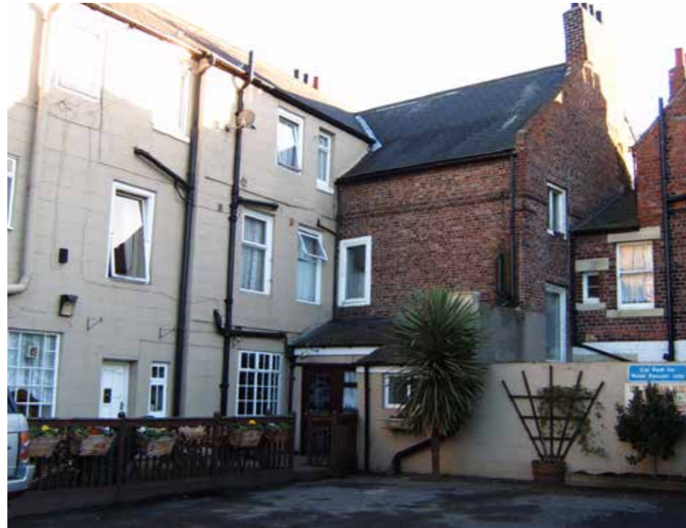
JUNCTION BETWEEN EARLY AND LATE GEORGIAN BUILDINGS
