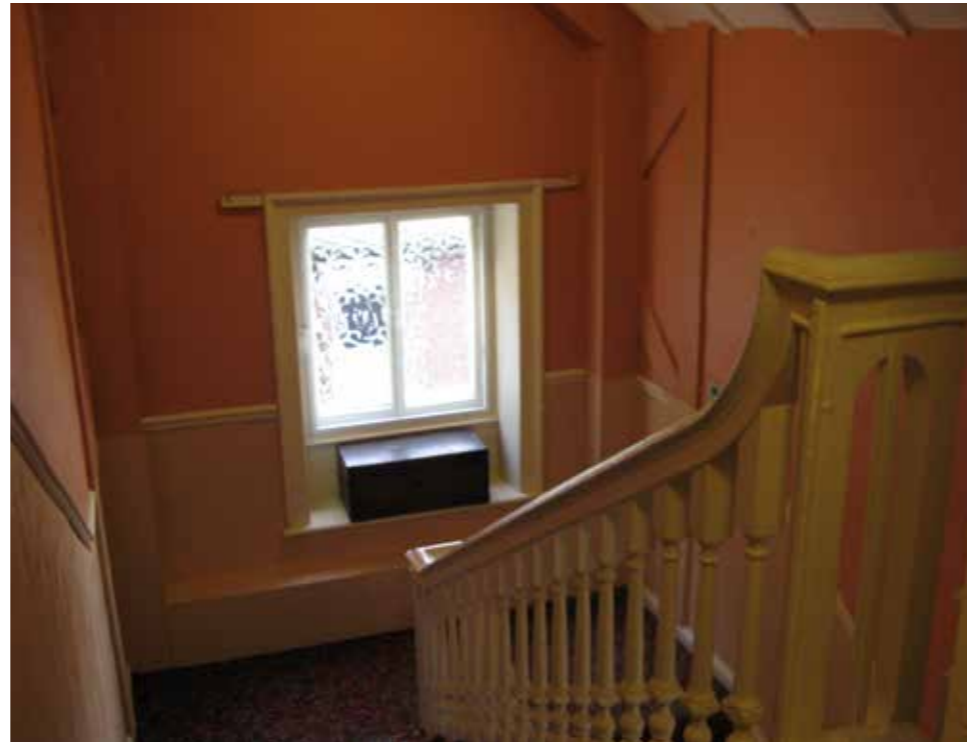
VIEW OF THE EXISTING STAIRCASE
