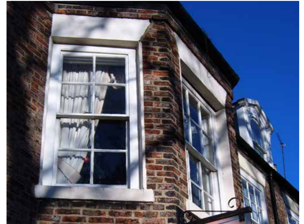
DETAIL VIEW OF THE EXISTING DOUBLE HEIGHT BRICK BAY WINDOW
