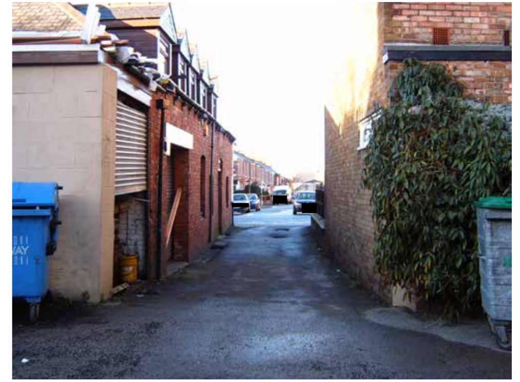
VIEW OF THE EXISTING VEHICULAR ACCESS FROM DEAN ROAD
